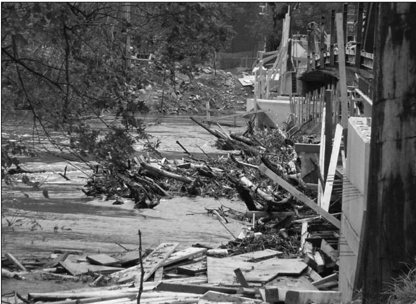
Figure 6. Debris at the Upstream Side of the College Street Bridge Source: Christopher Tomson.
