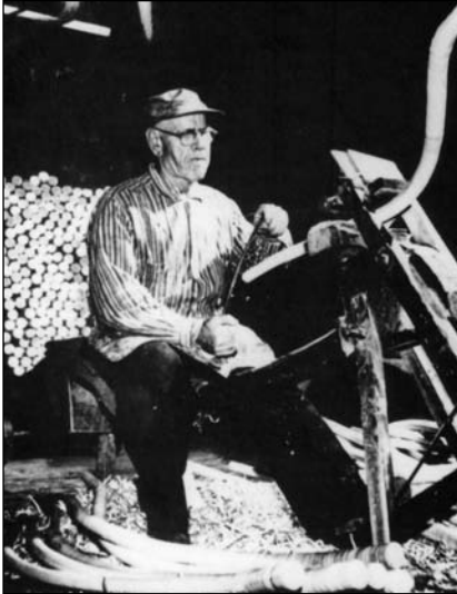
Figure 6. Preston (Pep) Ingham at work in the snath factory. Though many machines were used in the production of scythe handles, highly skilled employees nonetheless did a great deal of the work by hand. Ingham is pictured trimming flaws from all-but-finished snaths with a draw knife. His ingenious work bench incorporates a pedal which allows him to hold the sticks securely in place with his left foot, thus freeing both hands to shave away imperfections. Société d'histoire de Waterville, SR 740.
