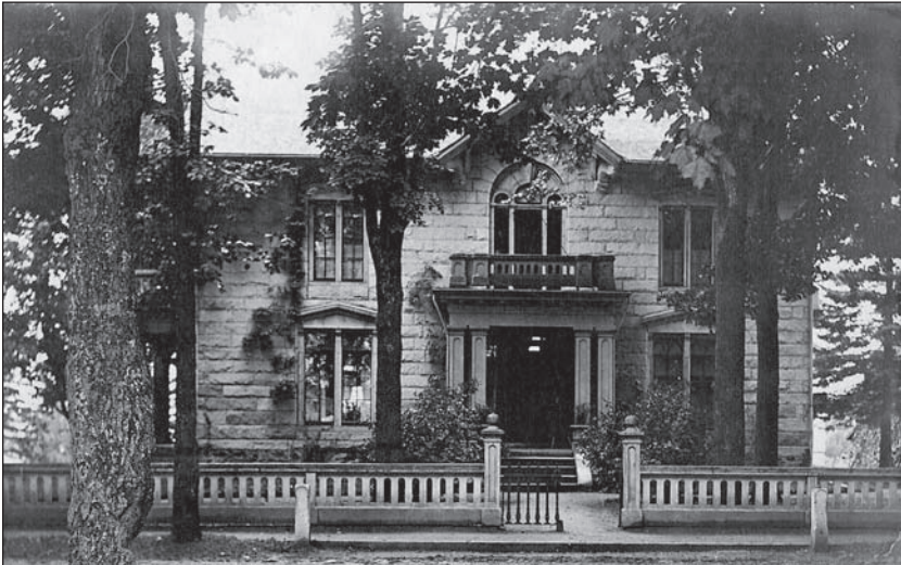
Fig. 1: The Colby house, 1859, was likely inspired by a model in A.J. Downing's popular pattern book Cottage Residences of 1842. The picturesque landscape and fence, shown here in 1905, were important features of Downing's vision. Courtesy of Colby-Curtis Museum and Archives.
