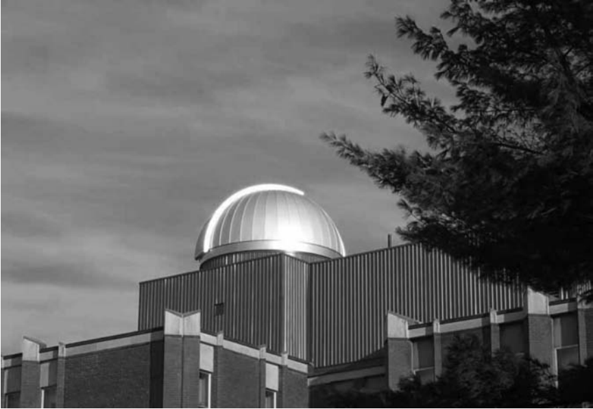
Fig. 4: The Bishop's University Astronomical Observatory on top of the roof of Nicolls building.
